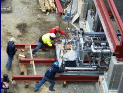
Sliding Skid Into Place on PRI-Engineered Rail System
