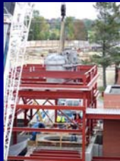
Lowering Vessel Onto Skid
