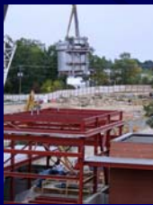
Lowering Vessel Onto Skid
